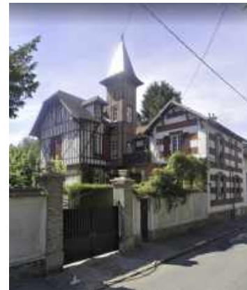
Villa, 63 avenue Gallieni
