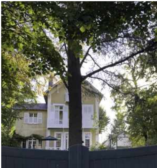
Villa, 27 avenue Gallieni
