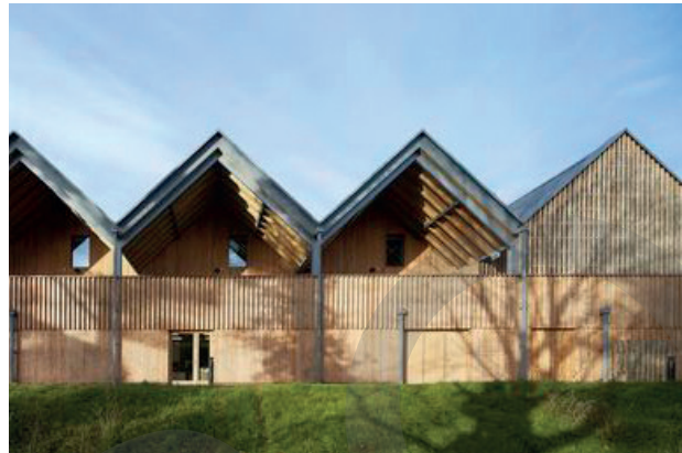
Bedales School of Art and Design Building / Feilden Clegg Bradley Studios © Hufton + Crow
